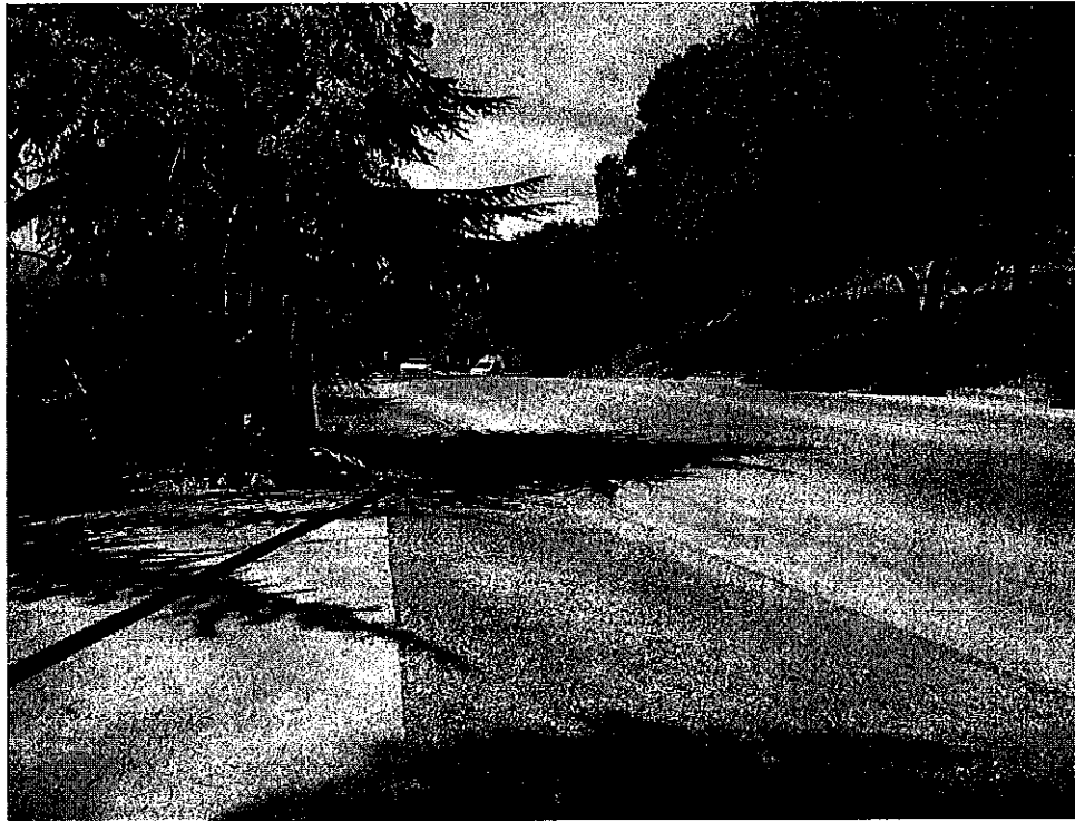
Figure 1 – Photo is taken from the Guidotti driveway, looking south on Stevens Canyon Road and the Residential Parcel. There is hump visible in the road here; approaching cars are seen to be downhill from the driveway. Due to an inadequate culvert/drain system, water from the ephemeral creek comes across the road and floods the Guidotti driveway during some storm events. Unless the hump in the road is reengineered, it seems very likely the Guidotti property will continue to flood during large storm events. Even with a new culvert/drain, the system is likely to be overwhelmed by the woody debris which the Guidottis say is common-
