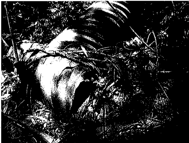
Figures 10, 11, 12 – Current outfall carrying storm water from ephemeral creek to Stevens Creek. The cement structure visible in bottom photo was installed circa 1946 and no longer carries water. The metal structure seen in the top and middle photos was installed sometime in the 1960's as part of system to drain the Residential Parcel after neighbors complained about the lake which had formed due to inadequate drainage.
